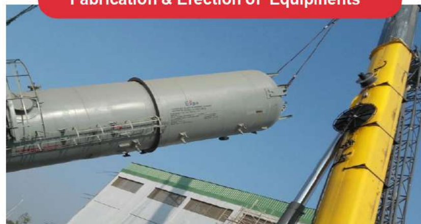
Fabrication & Erection of Equipments
